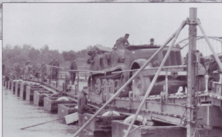
An Sd.Kfz. 8 halftrack of the 3. Panzer-Division crosses the Vistula River on a medium pontoon bridge (Brückengerät T). This 12-ton capacity vehicle was used as a prime mover for 15cm howitzers, 8.8cm and 10.5cm antiaircraft guns, and bridge section trailers.
