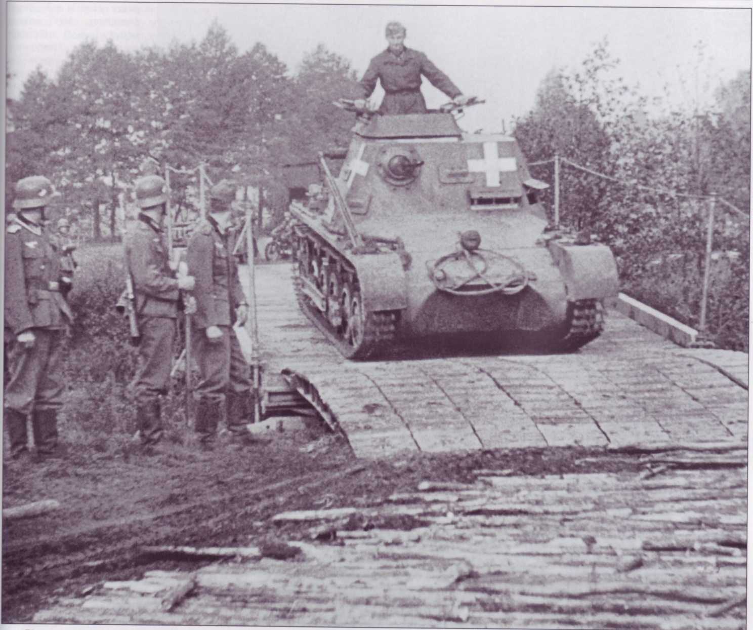
Pioneer troops stand beside their recently completed prefabricated bridge as a Sd.Kfz.265 small armor command vehicle (Befehlspanzer) crosses. The six 4-meter assault bridge equipment (Brückengerät) sections, carried by pioneer units aboard truck and halftracks, provide the off-ramp on to a corduroy road (log matting laid across a dirt road to prevent it from being churned into mud). Many tanks were painted dark gray overall, but a dark brown "cloud" camouflage pattern was also used of about one-third brown coverage. In black and white photographs it is often difficult to discern these two-color camouflage patterns.
